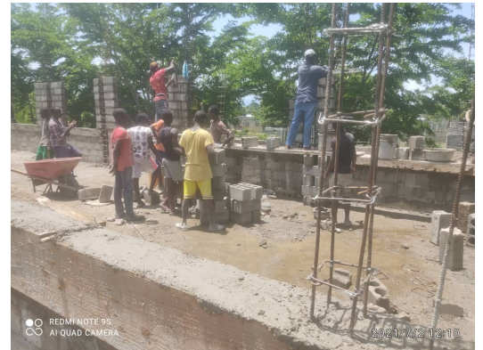
Construction Project at the school complex.
