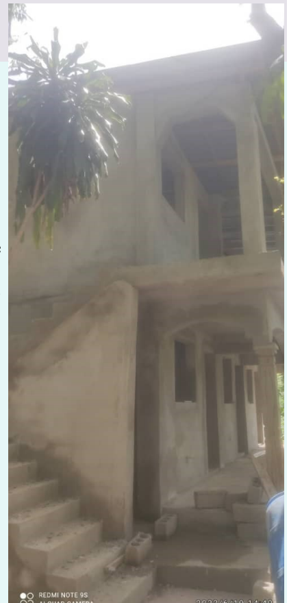
A new office is being completed at the boys Ophanage
