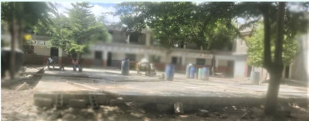
Concrete slab work at the School
